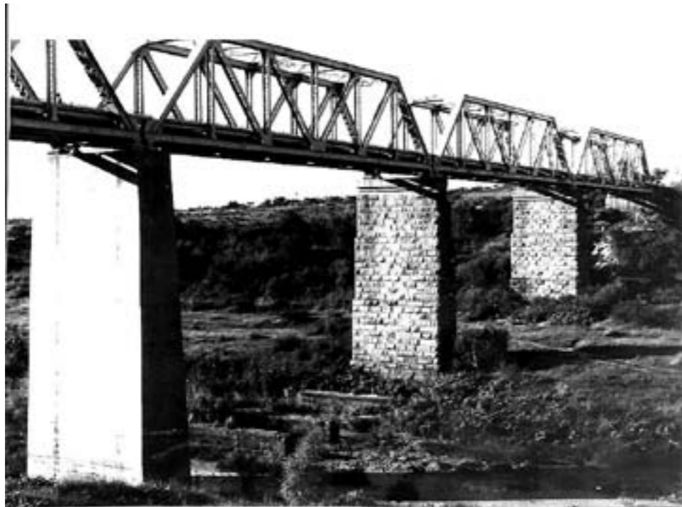
Bridge: Valsch river bridge (then)
